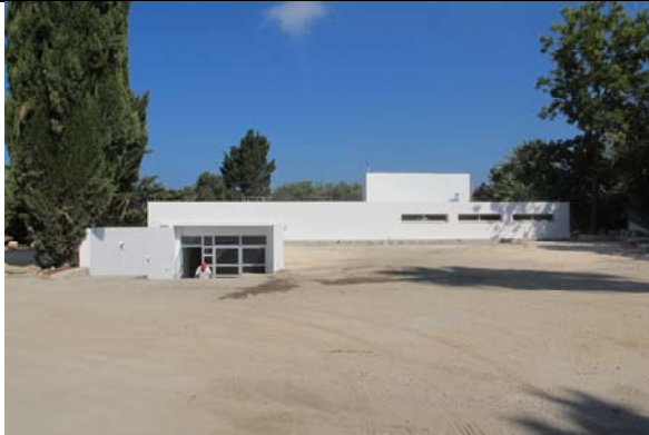
1. View from the parking area
